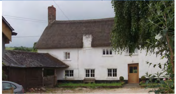
Figure 33 (above): East Holme and East Holme Farm
