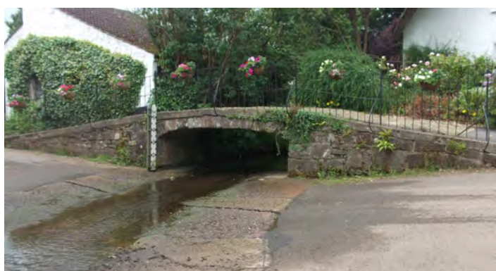
Figure 2 (above): Footbridge over ford, Pump Street
