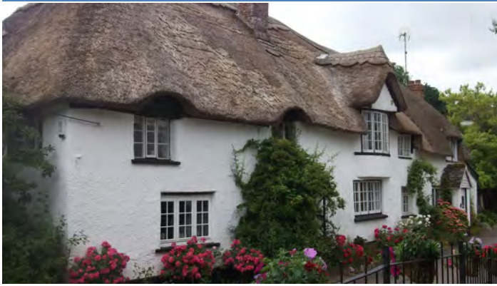
Figure 5 (above): Old Beams, Pump Street
