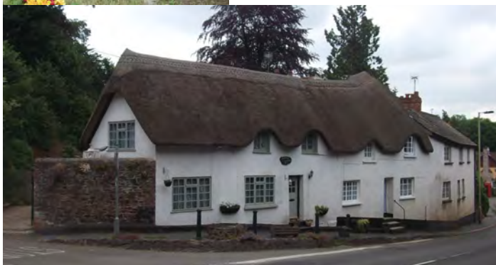
Figure 31 (right): The Forge and 33 The Village, Pump Street
